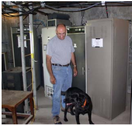
Figure 3 – Kim, WA1PBU, confers with the work party's security officer, Lucky. All of the club repeaters are visible in the background. From left to right: 6m, 2m & 220 MHz, 440 MHz, and 900 MHz.
