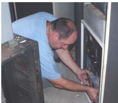
Will, N1PXA, installing the new dual-mode 64 repeater.
